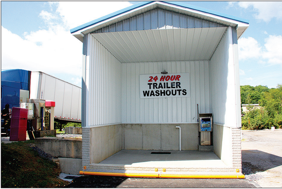
The new self-serve trailer washout bay at Hurricane Truck Wash.
