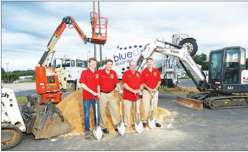
Stefan Pies, Henning O. Bruns, Bob Riley, and Joel Demelza break ground on a new logistics center at the Cleveland, N.C. Truck Plant.
