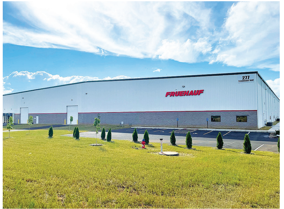
Fruehauf Dry Van Manufacturing Plant, located in Bowling Green, Kentucky.
