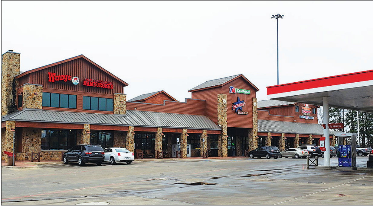
The new TA Express in Kilgore, Texas.
