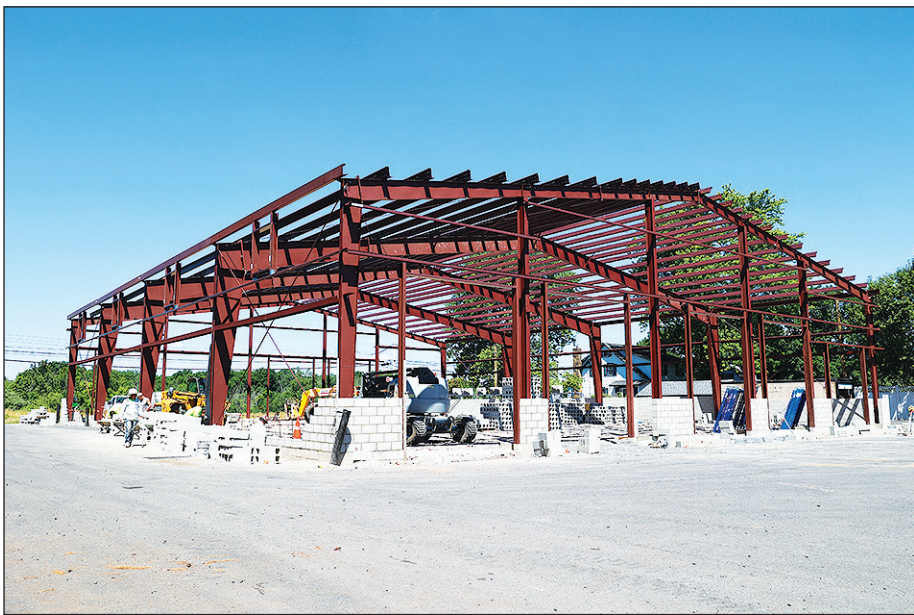
Vanderlely's new building under construction.
