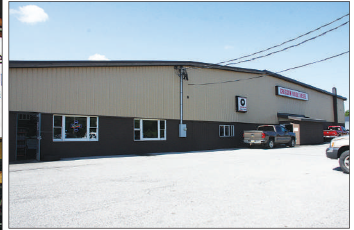
Cresson Ridge Diesel Garage
